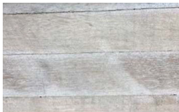
Small cracks due to temperature & humidity variations.
