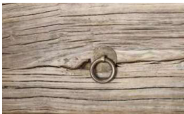
Small cracks along the grain line.
